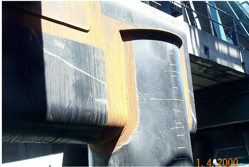
Figure 2. Typical Pile to Headstock Connection Prior to Touch-up Painting
