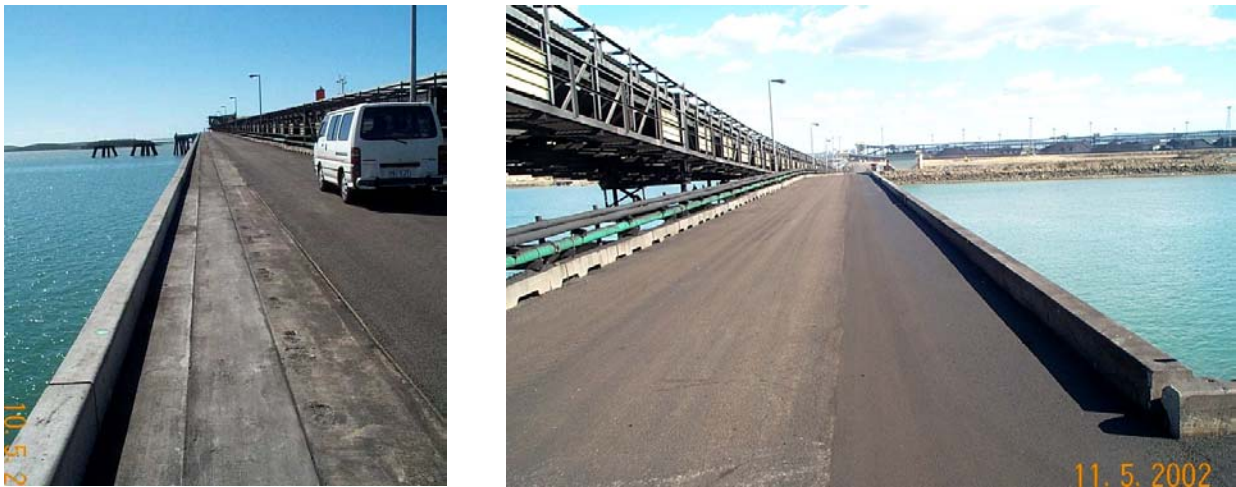
Figure 5. Jetty Widening Before and After Asphaltalting
