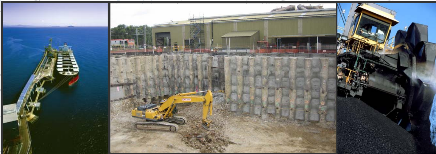
Excavation and civil works for the new Rail Receiving Station
